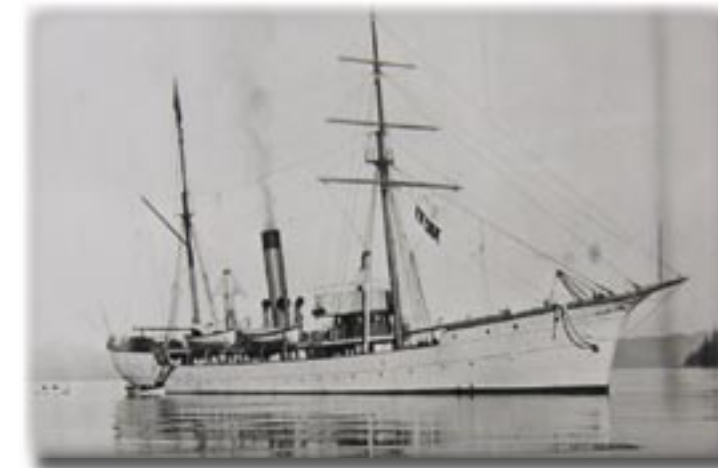
Albatross- Alaska's Pioneering Research Vessel Built in 1882 on the Atlantic coast, the iron twin screw steamer was 234 feet long and 384 tons. She was rigged as a brigantine. She moved to the Pacific in 1888 for the purpose of marine surveys and made annual trips to Alaska for over 20 years. She helped collect information on the sealing industries and cod first and later turned to salmon. In 1892, the fisheries research vessel was assigned to patrol the Bering Sea and was mounted with a revolving cannon. In 1897 she was commanded by Moser for the chief purpose of salmon research. The Albatross met her end when she went on the rocks in bad weather while trying to enter Lituya Bay. Photo courtesy University of Washington Libraries, Special Collections, Cobb 3121.
